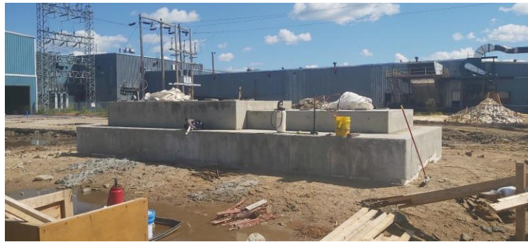
07-06-2020 – Forms on Turbine Foundation Stripped
