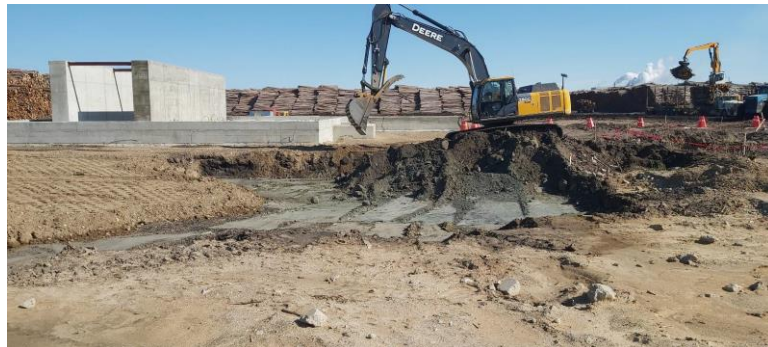
07-16-2020 – Waste Removal During Site Groundworks
