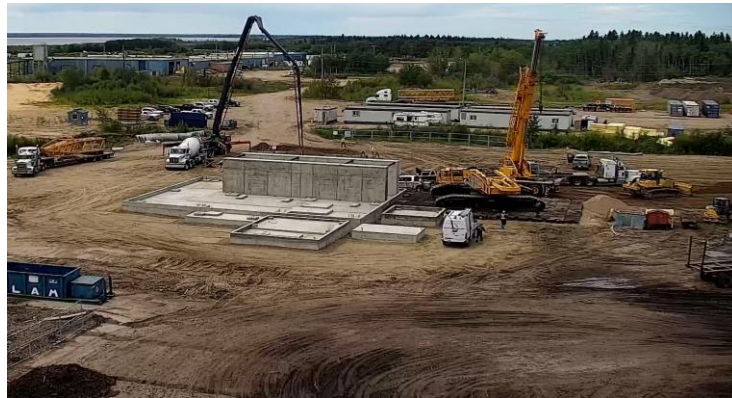
08-26-2020 – Crane assembly well underway
