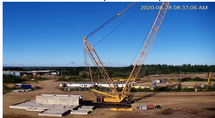
08-28-2020 – Crane mobilization complete.
